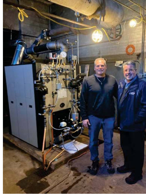
Joe Sestitio & Charlie Uglietto from Cubby Oil with the new furnace
